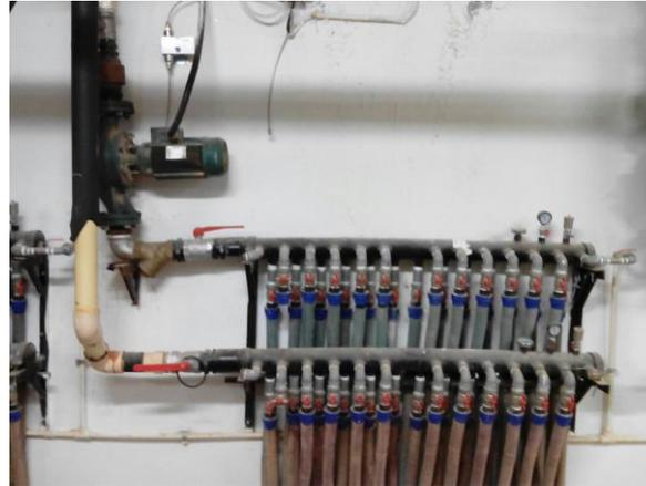
Photo 3: Source collectors (bottom) and Return collector (top) at AUM with AAV, pressure gage and Temperature gage
