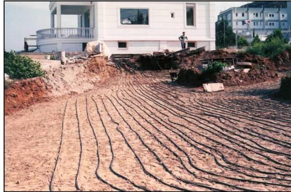
Photo 1: Horizontal loop for heat exchanger
