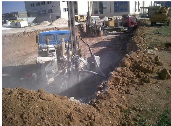
Photo 2: Construction of the AUM geothermal system (Vertical heat exchanger)
