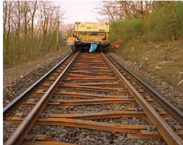
Figure 2 Y-Steel-Sleeper [23]
