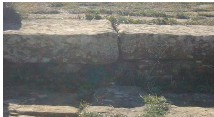
Figure 6. Section in the structure of a route through the city of Timgad
