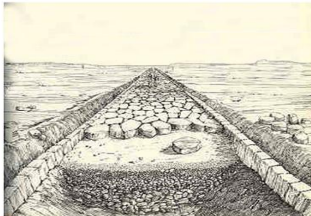
Figure 5. Implementation of a road
