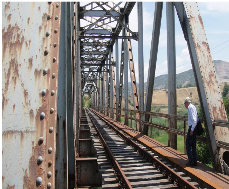
Figure 1. Internal view of the old steel truss Railway Bridge
