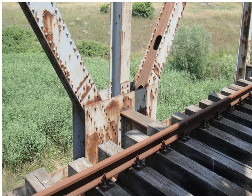
Figure 2. View of a main truss-deck riveted joint of the bridge
