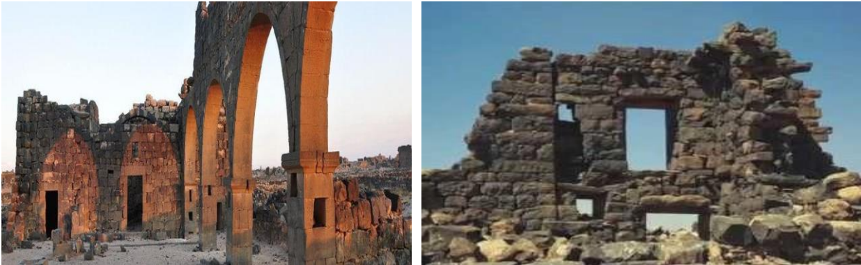
Figure 2. Basalt rock as a building stone, the old city of Um Al-Jimal, Al-Mafraq district.
