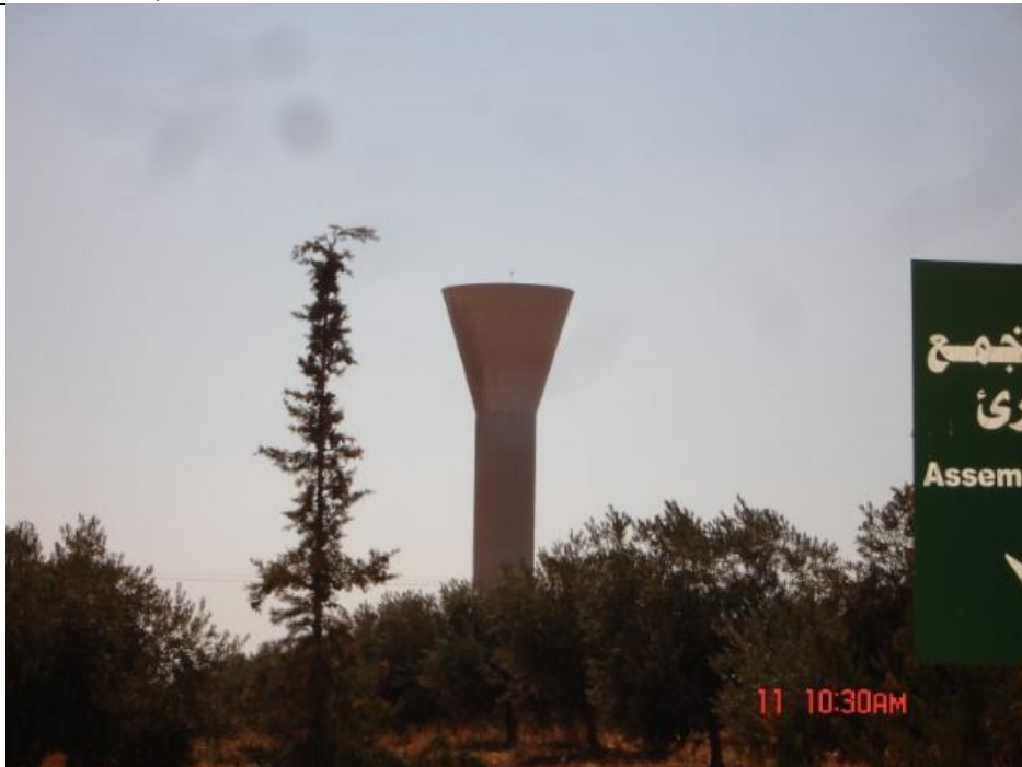
Example of Water Conservation - water tower tank (JUST, Jordan)
