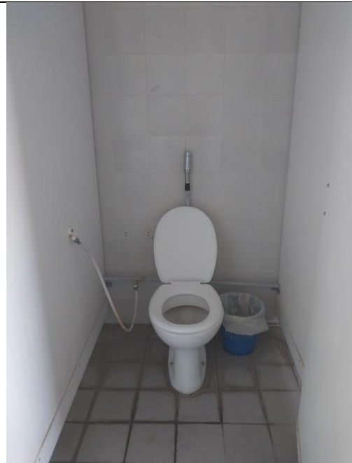
Due to the large density of university facilities users, and the severe pressure on health facilities, a flash valve system is used to clean toilet seats, and it is
