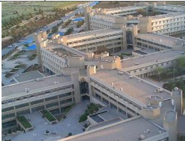
As shown in picture above the Engineering and Medical colleges buildings facades designed extroverted to the inside court, so the halls and laboratories are gain natural lighting and natural ventilation and avoiding direct sun heat,for acknowledgment there are fountain systems in each court that helps cooling the university surface, while the outer facades are mostly solid with small architectural openings to avoid most
